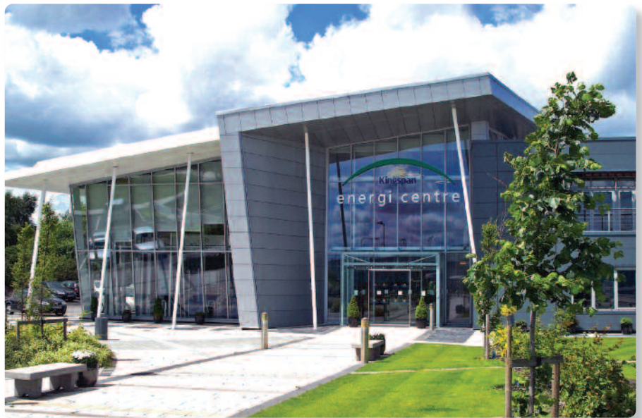
Kingspan's Energi Centre, Holywell, North Wales
