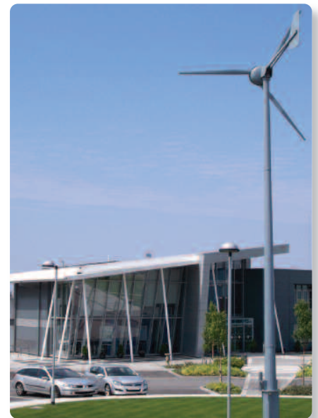
Wind turbine at Kingspan's Energi Centre, Holywell, North Wales
