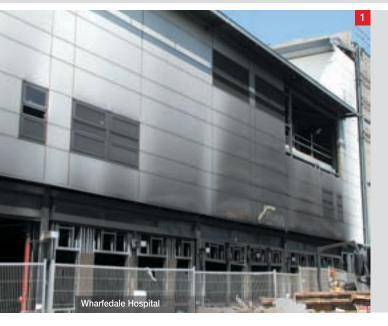
2 Sections were cut out of the short panels in order to inspect the steel column behind the panels. The photograph below left shows this more clearly. Close-up of the inspection holes cut in the panel after the fire. The insulation core can be seen clearly and
