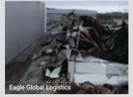
and flames generated by the burning building were so intense that the paint coating on the Kingspan panels on part of the next-door building was burnt off but the PIR core did not ignite and no flames or smoke entered the adjoining building.
