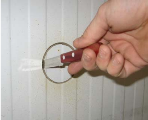
7. Using a long blade cut through remaining foam and foil
