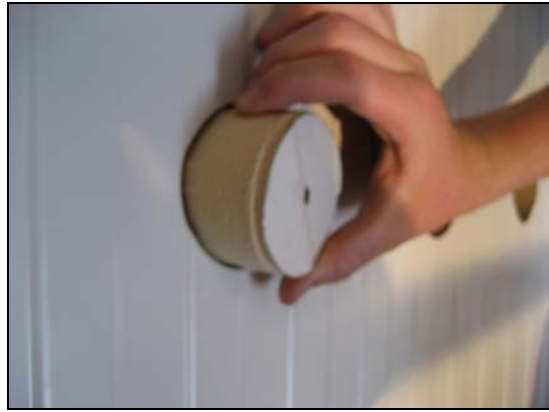
6. Remove cut piece from panel
