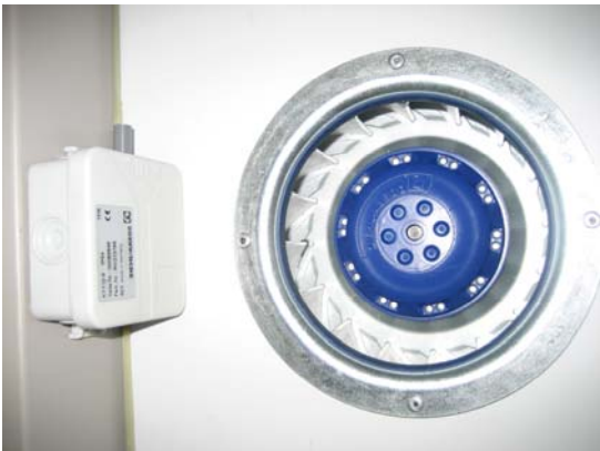
8. Place Temperature sensor inside plenum adjacent to fan inlet.
