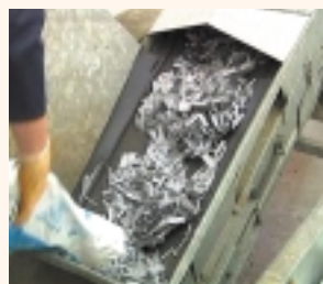
Steel fibres added to hopper
