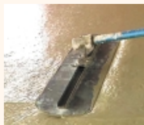
Floating provides a smooth finish
