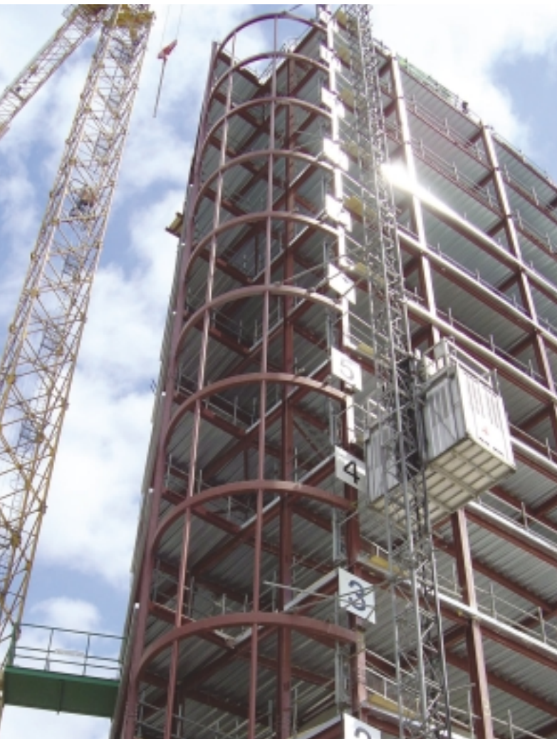
Two Towers, Arnhem, Netherlands. Photo Courtesy of MSW (UK) Ltd.
