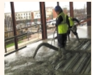
Mixture spread onto deck
