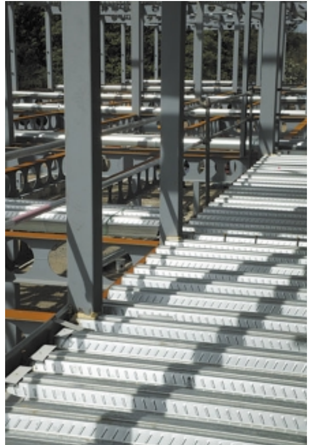
Completed deck layout from layout drawing opposite.
