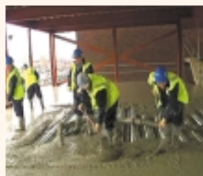
No mesh means no tripping hazard
