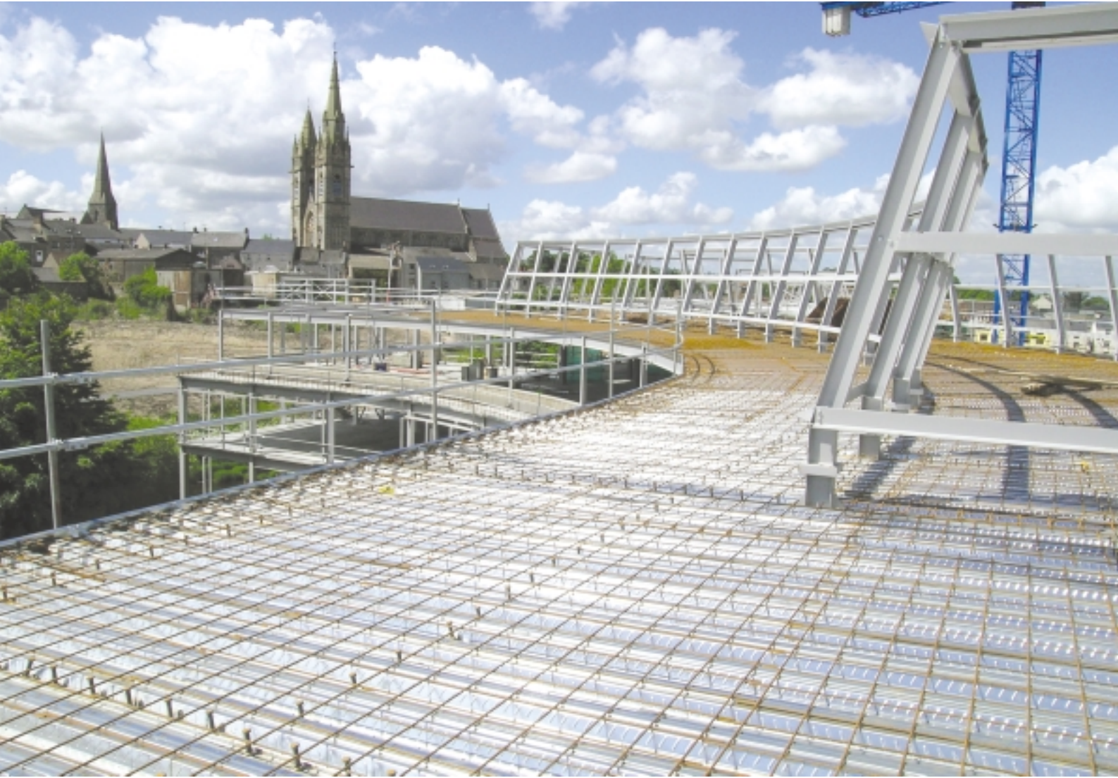
Multideck was used in the construction of Omagh College, Co. Tyrone. Photo Courtesy of Composite Design Ireland Ltd.
