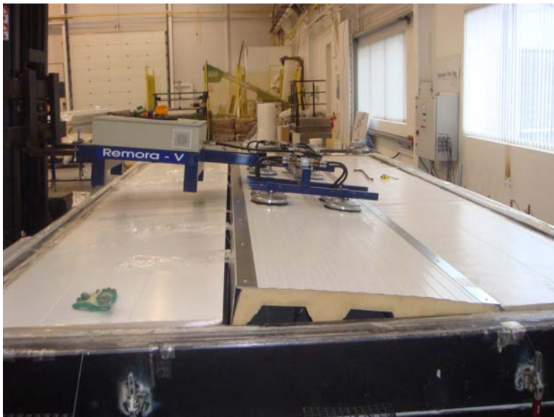
Figure 3.1: Floor-Dek panel with perimeter C sections lifted into vacuum rig
