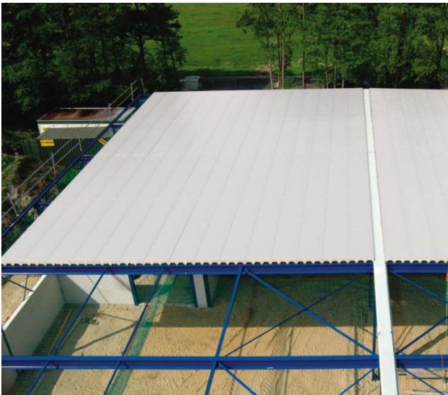
Figure 2.6 Floor-Dek used in long span roofing applications
