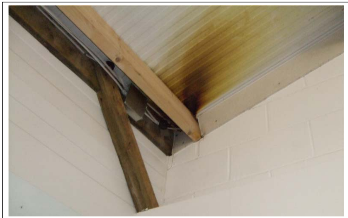
Figure11 - photograph of underside of roof in adjacent demise
