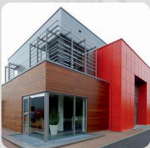
Arcomet , Beringen. Architect: Buro A-Ateljée, Prosper Baelen, Beringen.
